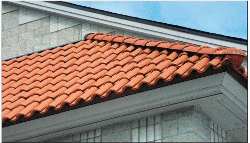
Tile installation was a blend of Old and New World techniques.
